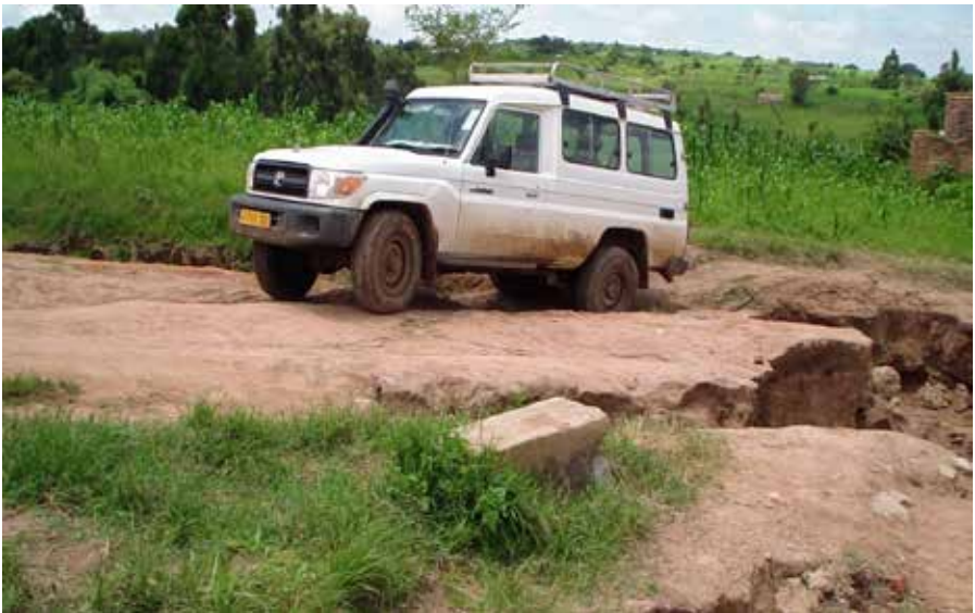
Picture 13: HAKIARDHI member Mr. Abdallah Matata looking for a place where the motor vehicle will pass to Kisasa villages due to heavy rainfall which deteriorate the road.
